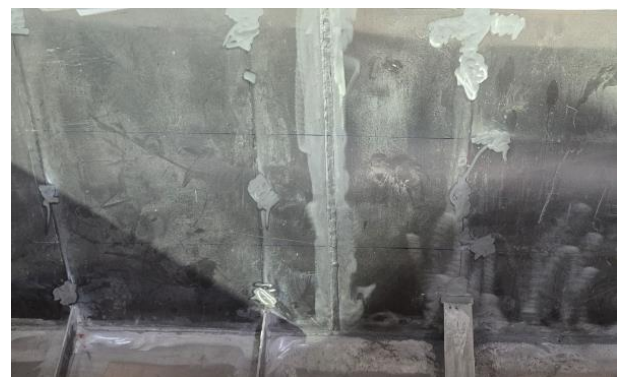
Figure 5. Welded joint image at the internal region of the transom Source: author
