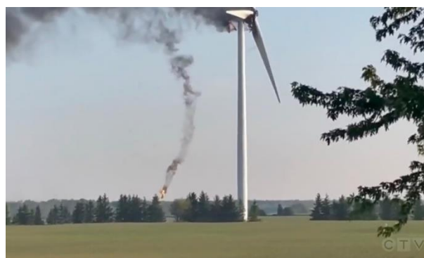
Figure 1. Wind turbine fire (Kingsbridge 1 2024-06)
