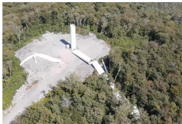
Figure 2. Tower collapse (Bow Lake 2021-08)
