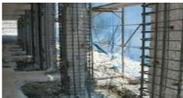
Figure 15. Lining of reinforced concrete columns
