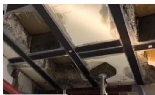
Figure 19. Floor reinforcement with CFRP composite material
