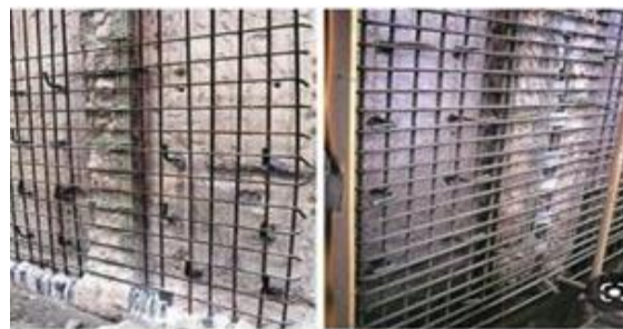
Figure 16. Lining of reinforced concrete walls
