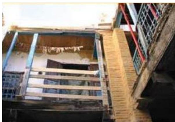
Figure 3. Rebuild of a traditional masonry pillar
