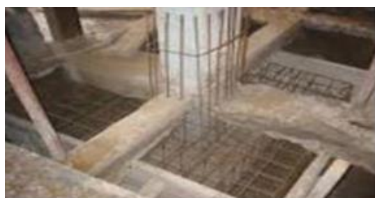
Figure 11. Lining of reinforced concrete footing
