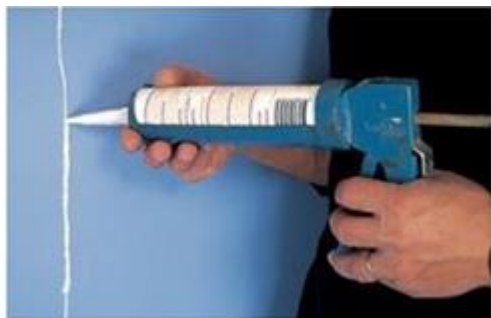
Figure 21. Repair of Cracks in Wall with Epoxy-Based Coating
