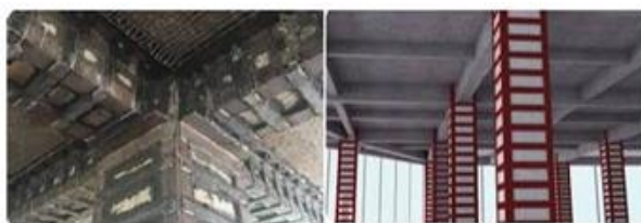
Figure 13. Lining by welded angles and flat iron
