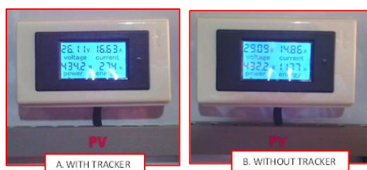
Figure 16. Power Generation of the PV Module at 1PM (With Tracker vs Without Tracker)
