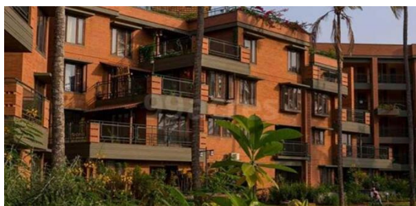
Figure 4. Malhar terraces Open terraces
