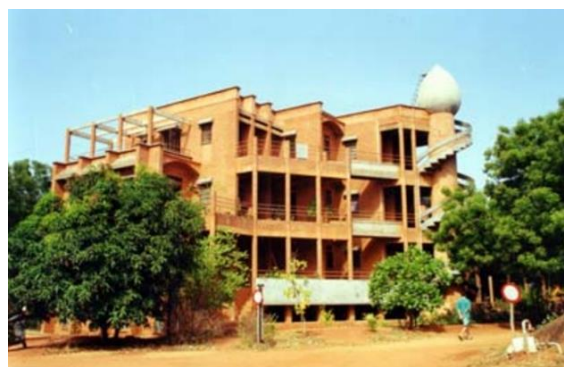
Figure 1. Vikas Community third building block
