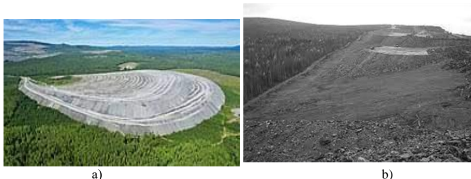
Figure 1. Placement of overburden rocks, a) dumps on the horizontal surface (photo by Vyacheslav Bukharov), b) on the inclined surface (photo from Shpakov and Yunakov, 2018).
