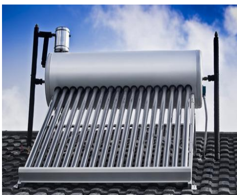
Figure 9. Evacuated tube Solar Collector (Sandeep et al., 2016).
