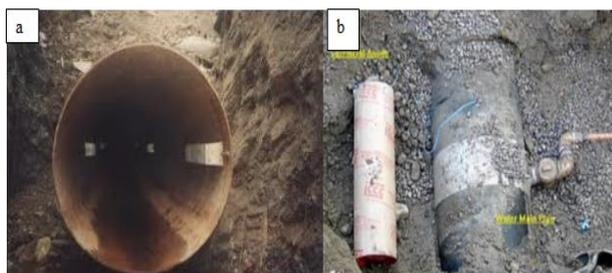
**Figure 10.** (a) Internal protection of water pipe-line using sacrificial anodic method (b) External protection of water pipe-line using sacrificial anodic method
