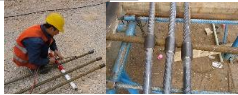
Figure 27. Three samples of rebar couplers type A prepared for tensile test
