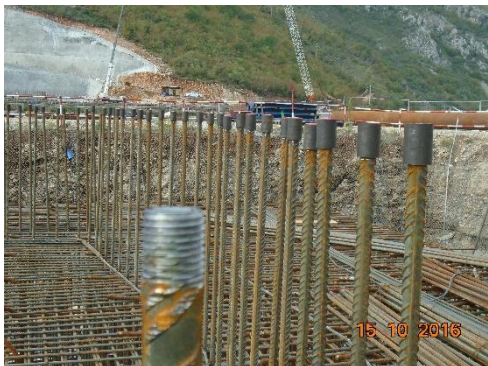
Figure 15. Threaded reinforcing bars in foundation which was continued by mechanical couplers
