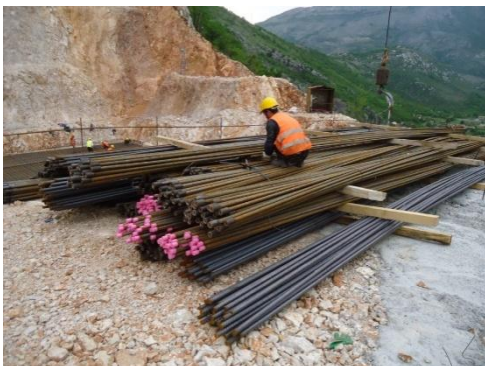
Figure 21. Threaded bars stored on the site
