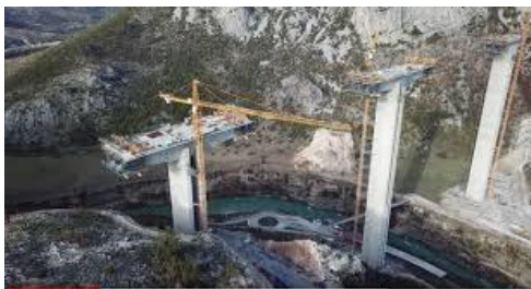
Figure 10. View on the bridge Moračica
